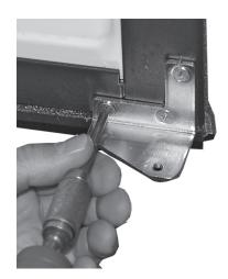
7. Remove the plugs that cover the screw holes located on the opposite side of the present hinge location.
